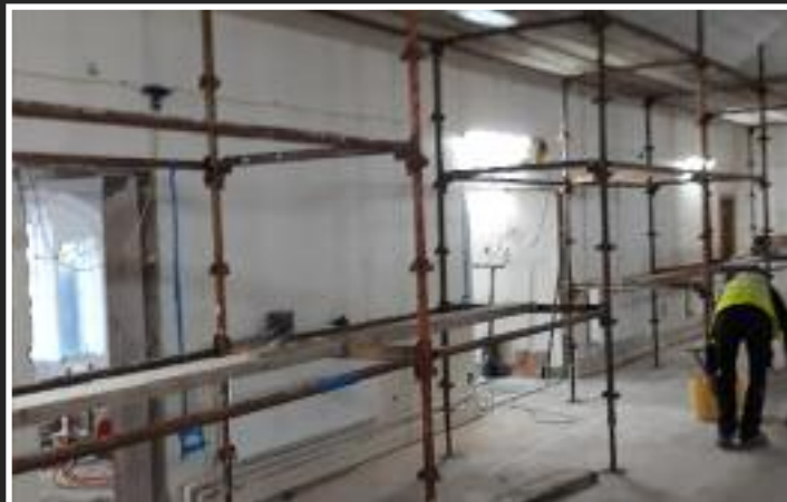
Renovations to Caledon Parish Hall.
